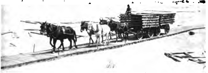
Hauling sections of plank road out into the desert on the El Centro-Yuma Highway.
